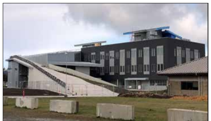
Figure 6: The Gladys Valley Marine Studies Building in Newport, Oregon is designed and built to sustain a magnitude 9.0 earthquake and the ensuing tsunami. The 47-foot ramp leads to the roof of the three-story structure, which is designed to serve as a vertical evacuation site for more than 900 people.
