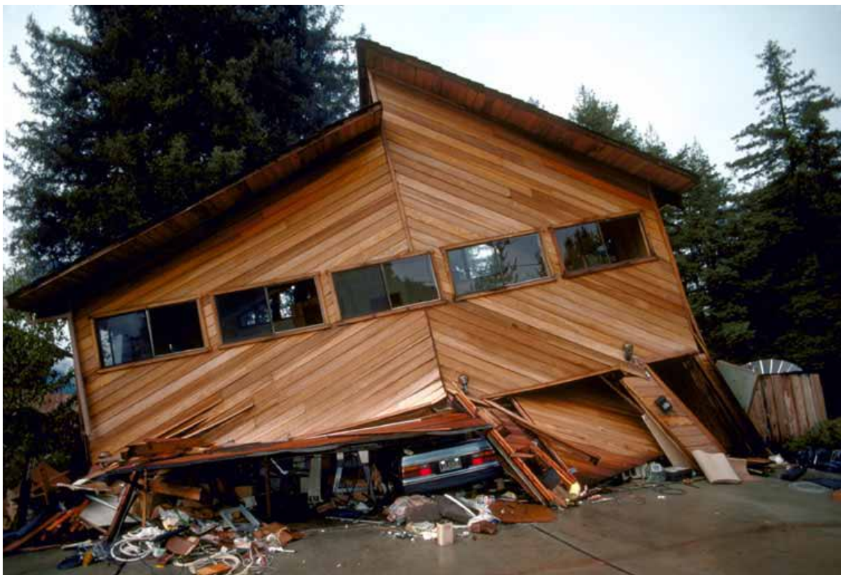
Soft first floor garage, lacking shear strength, causes house to collapse during strong shaking. Image source: U.S. Geological Survey
