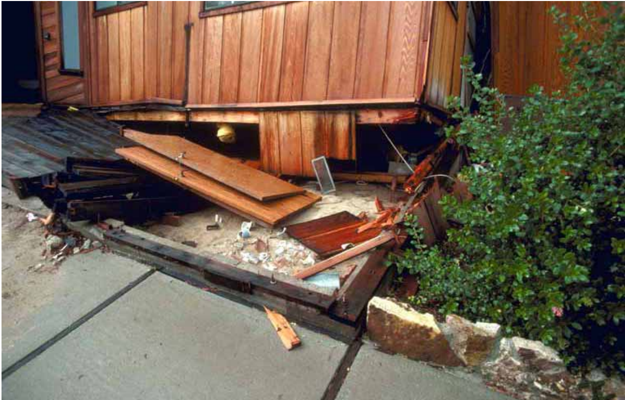
Cripple wall lacking shear strength contributed to house collapse. Image source: U.S. Geological Survey
