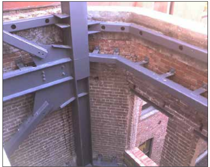
Figure 5: Structural reinforcements showing gussets, steel bracing and moment connections in an unreinforced masonry building. Image source: Dave Mathews
