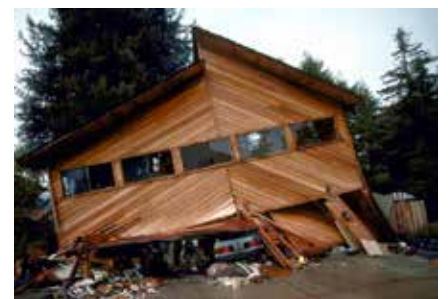
Figure 2a: Soft first floor garage lacking shear strength collapsed house.
