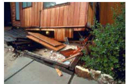
Figure 2b: Cripple wall lacking shear strength collapsed house.
