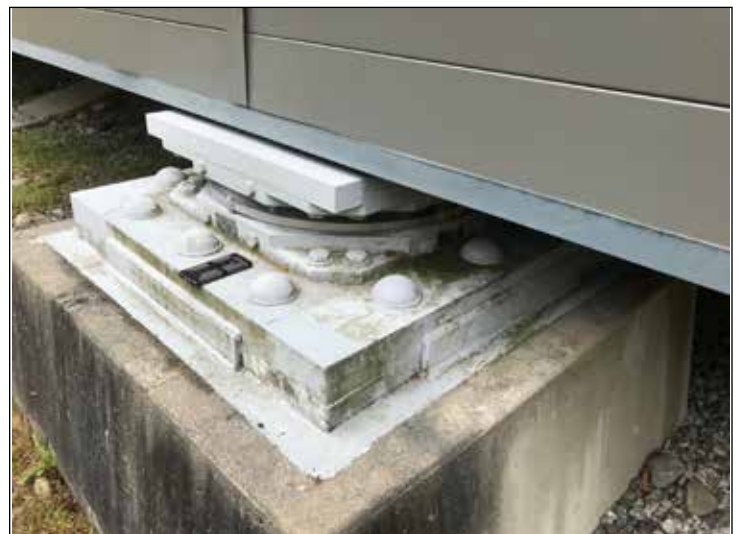
Figure 6: Base isolators at the Washington Emergency Management Division building. Photo courtesy of Washington State Military Department Emergency Management Division
