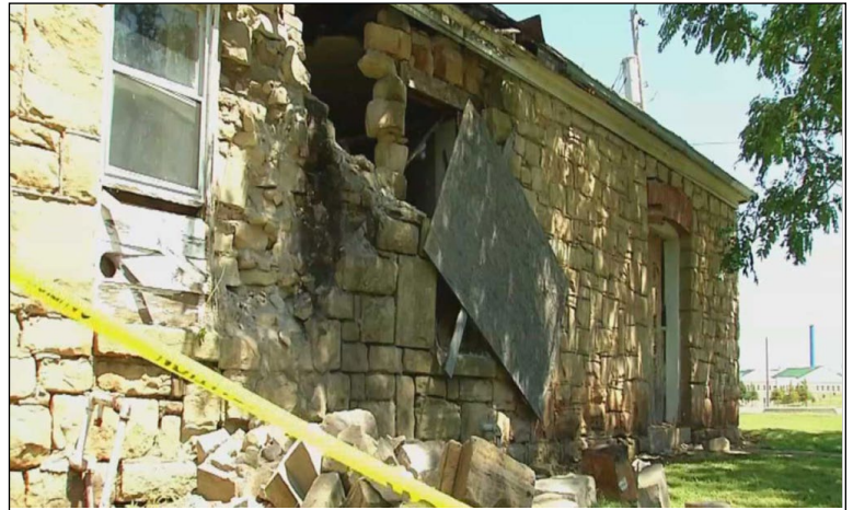
Figure 1. The sandstone façade of this 100-year-old historic building in Pawnee, OK was damaged due to a M 5.8 earthquake that occurred nearby on Saturday, September 3, 2016. (Photo: Oklahoma Channel 9 News)
