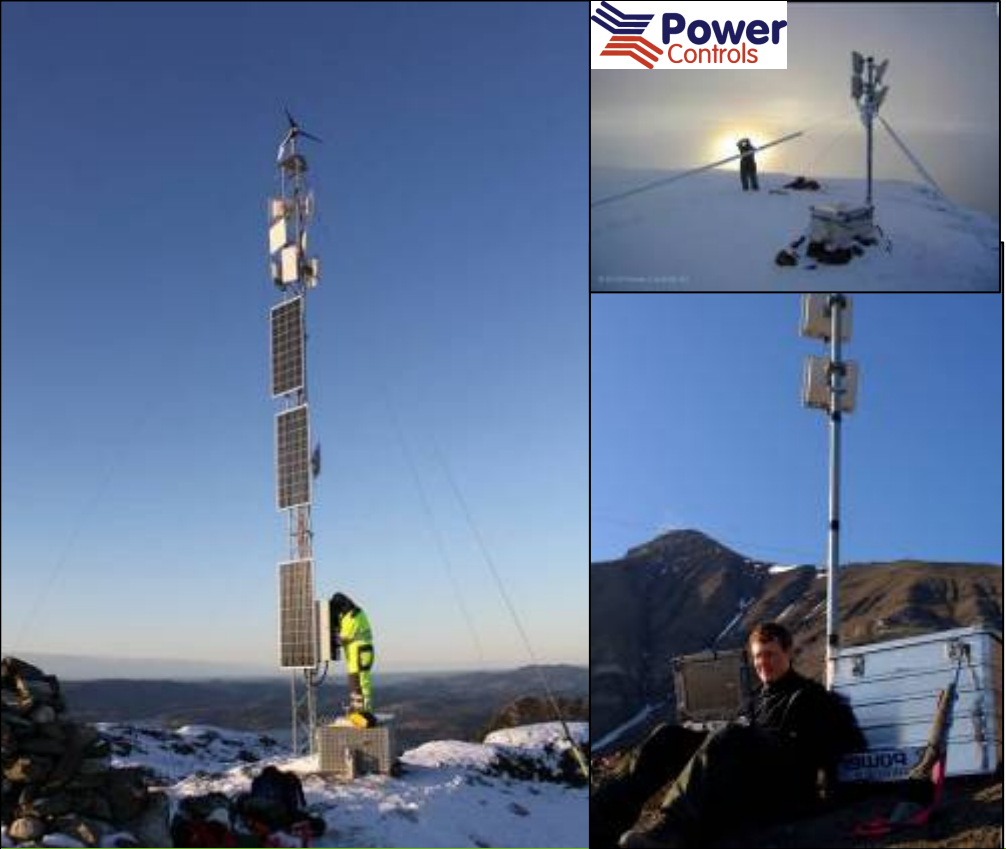
Repeater Stations EFOY Pro in Insulated Outdoor Box (Norway)
